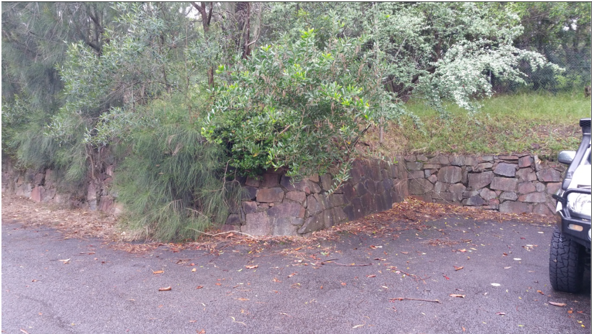
Figure 5: Existing Rock Retaining Wall along Eastern Site Boundary
