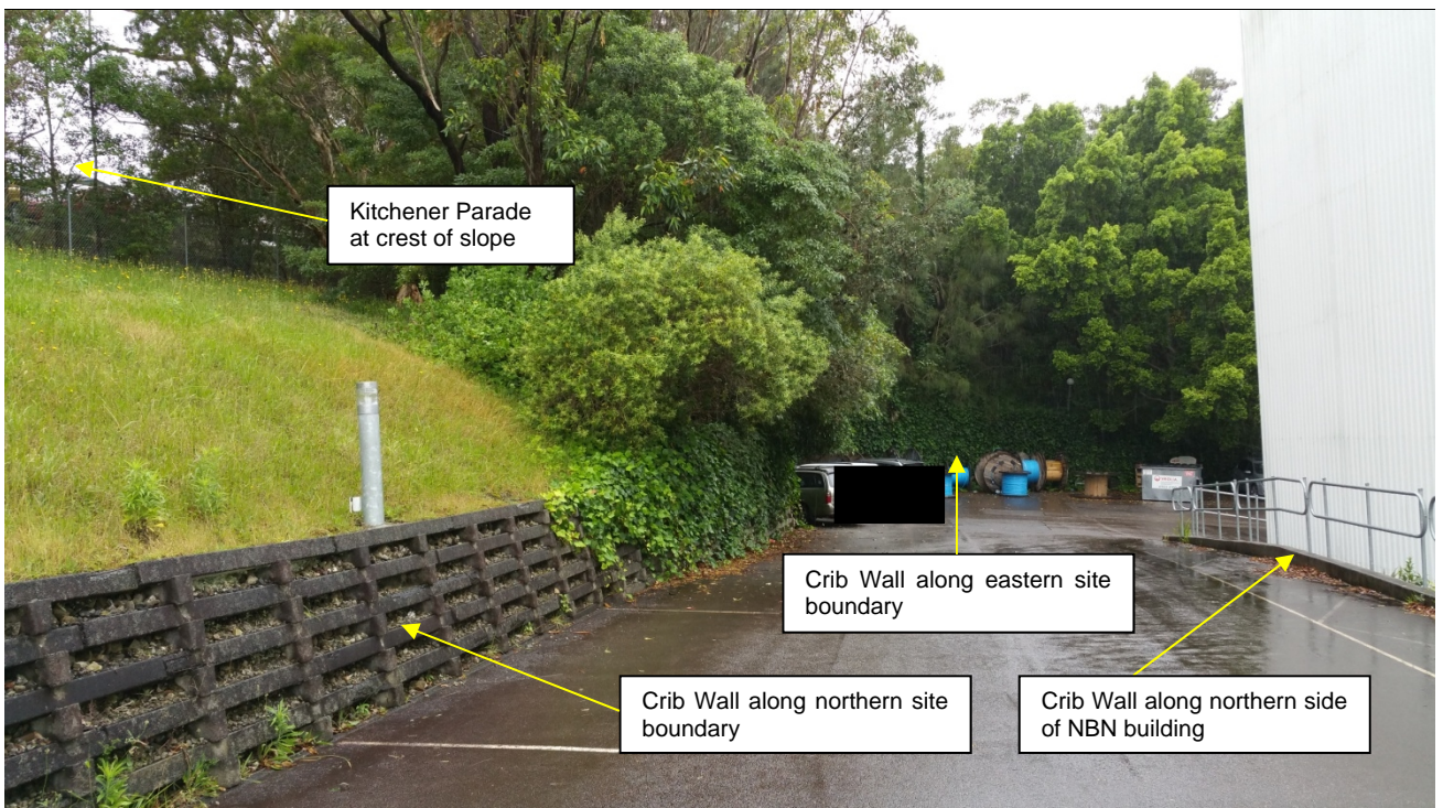
Figure 6: Existing Crib Retaining Wall along Northern Site Boundary (looking east)
