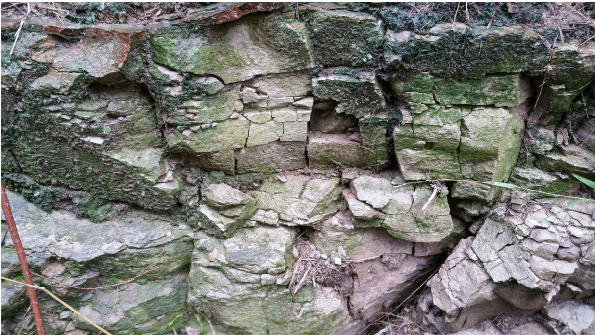
Figure 7: Exposed Siltstone along parts of eastern boundary (adjacent to air conditioning containers)
