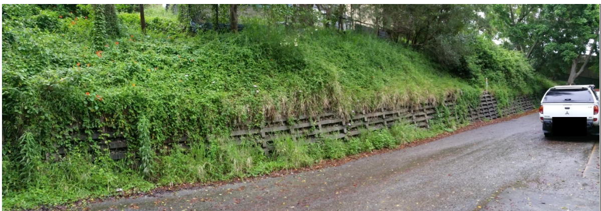
Figure 4: Existing Crib Retaining Wall along Southern Site Boundary (looking west)
